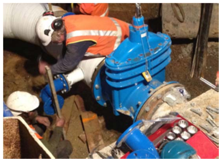
New valve to connect with the 100 year old sewer
