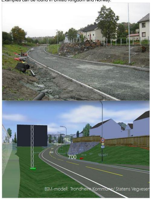
Figure 8. Road construction and accompanied BIM-model of same road in Trondheim (Norway)
