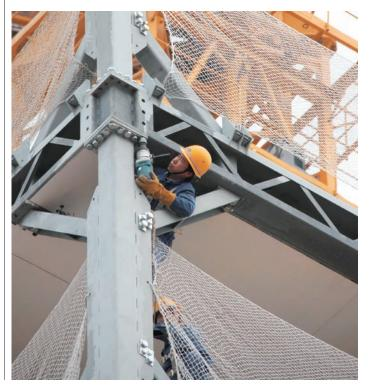
Previously, such honeycomb steel, being very costly to produce, was limited mainly to aerospace design, but BSB succeeded in bringing down the cost dramatically by inventing automatic copper-brazing streamline production. The company also uses the innovative steel for columns, crossbeams, floor slabs, walls and roofs.
