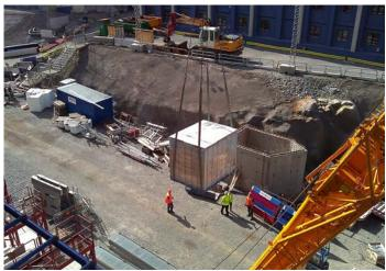
hotel construction, but had never before been used in hospital construction). Prefabrication has been applied to other components too, and helps to reduce manual labour and avoid the need for scaffolding; prefabricated mechanical and electric modules, for example, are simply lifted to ceiling level and welded together in situ, and prefabricated structural concrete elements and façade modules are simply lowered into place by cranes.
